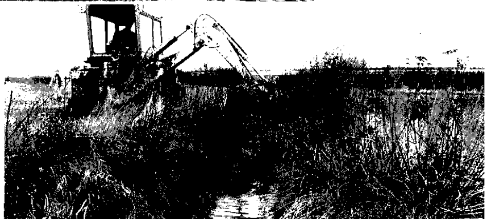
Dredging a watercourse
