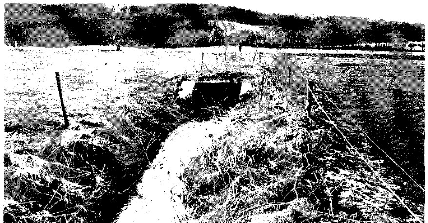
Figure 4.2 Many watercourses are interrupted by culverted sections.
