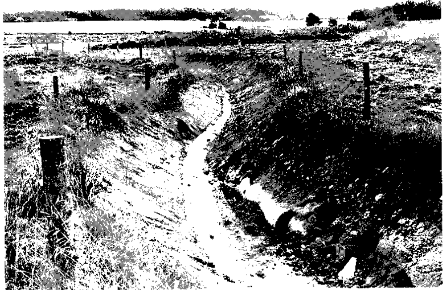
Figure 4.13 Enggård Bæk brook; formerly culverted, now open and meandering.
