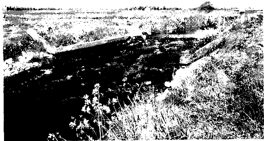
Figure 4.16 This is how weirs were modified in Sønderjylland in 1993; they were broken up and replaced by riffles.
