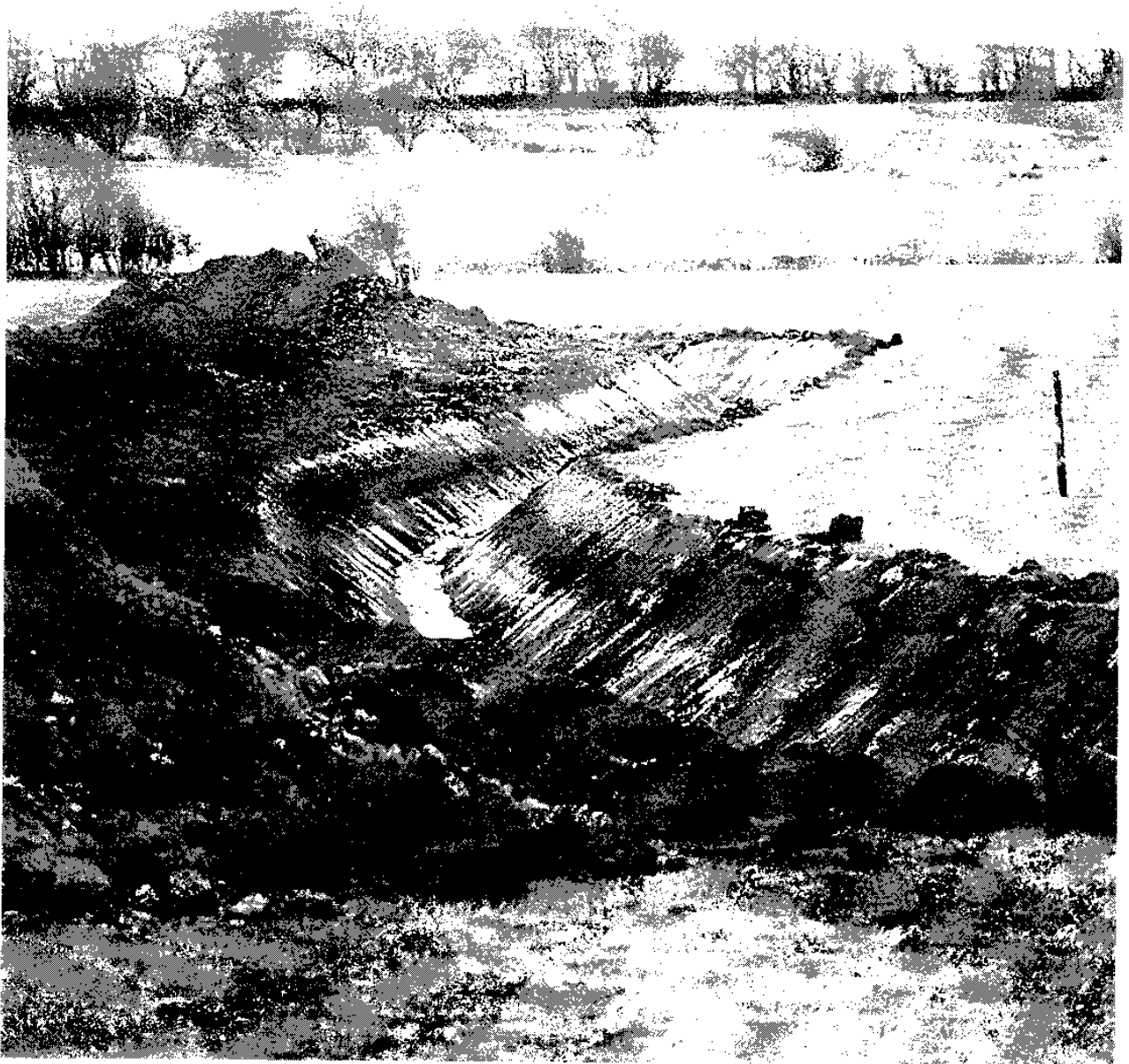
Figure 4.9 A meandering brook was excavated alongside a culverted section of Isholm Landgröft brook. Photograph by Frank Eliasson.
