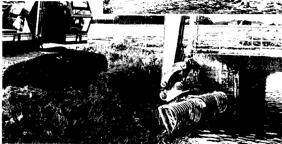
Clearing weed using a basket reaper
