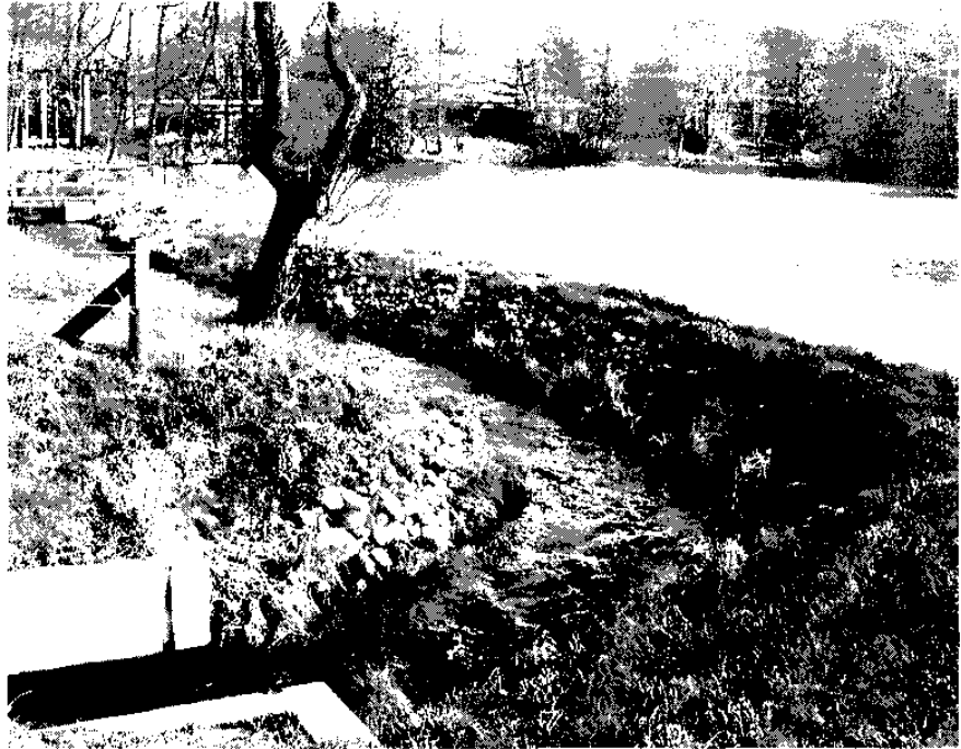
Figure 4.20 Bypasses are a good solution for passes at dams. Here is a well-functioning bypass in the river Skjernå.
