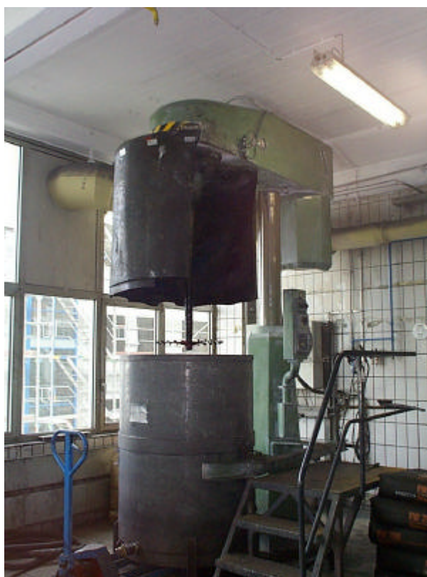
Photo 6: Encapsulation of dissolver with mobile bin and exhaust air extraction.
