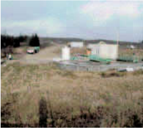
The leachate from the landfill at Kaunas is collected and treated as part of the DANCEE project at "Lapes landfill".
