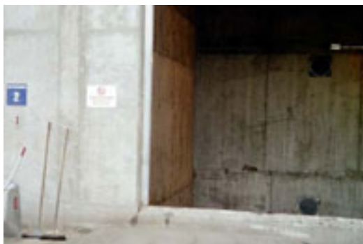
Figure 6.7.4 Hazardous waste bunker, NORCEM, Norway, August 2002
