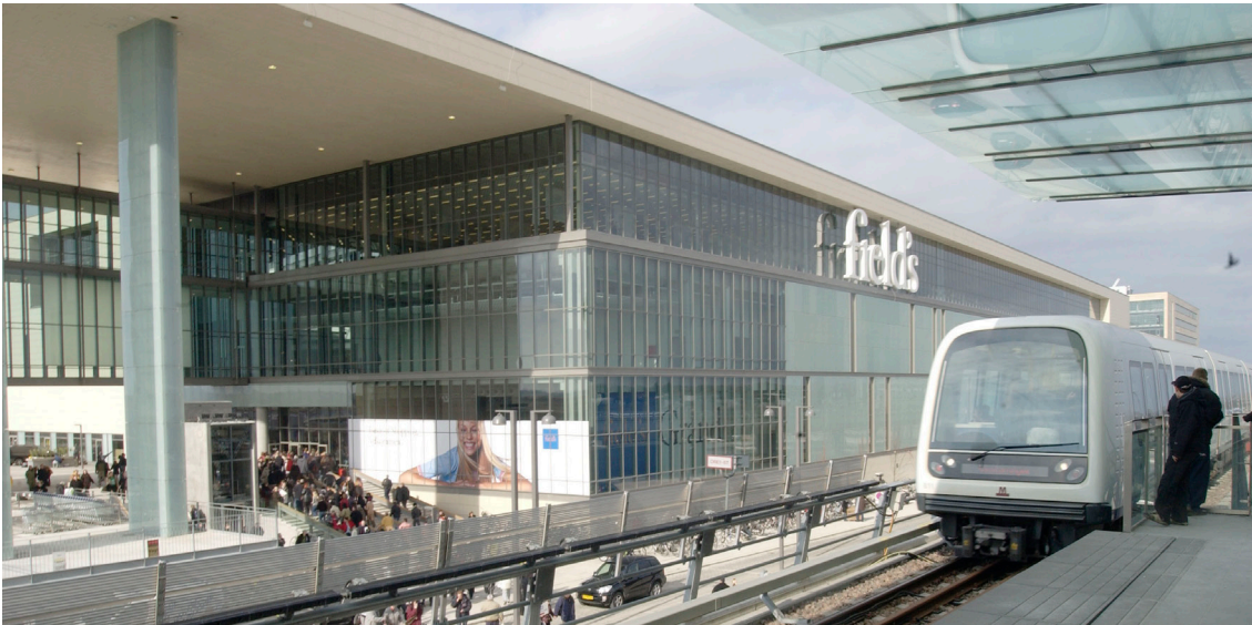
Photo 7: The shopping mall “Fields” in Copenhagen is cooled by ammonia chillers.
