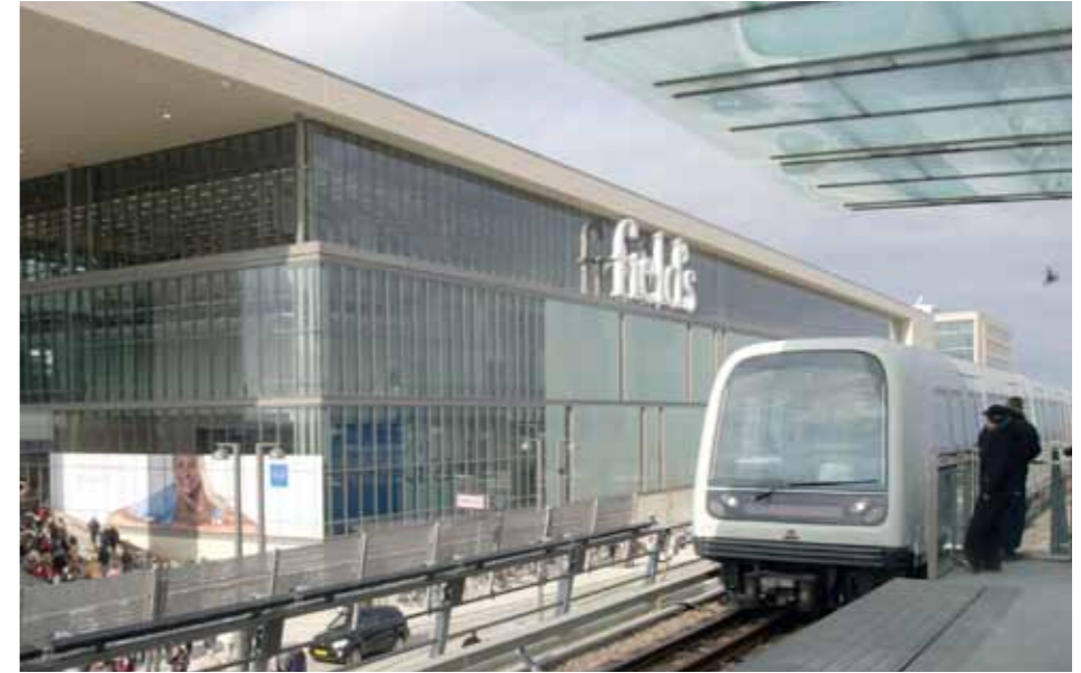
The shopping mall “Fields” in Copenhagen is cooled by ammonia chillers.
