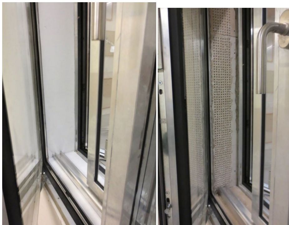
Illustration 8M. Photos of the applied absorber. Left side: 20 mm SUND ®. Right side: Perforated plasterboard plate in front of mineral wool in the wall cavity.
