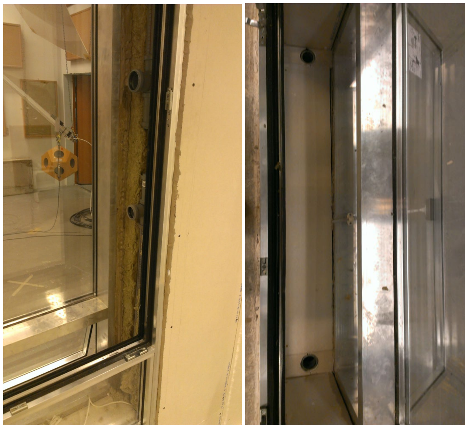
Illustration 7D. Photos of the window with inserted resonators. The Left photo depicts the resonators mounted in the vertical frame, while the right photo shows the resonators mounted in the horizontal frame (the bottom).
