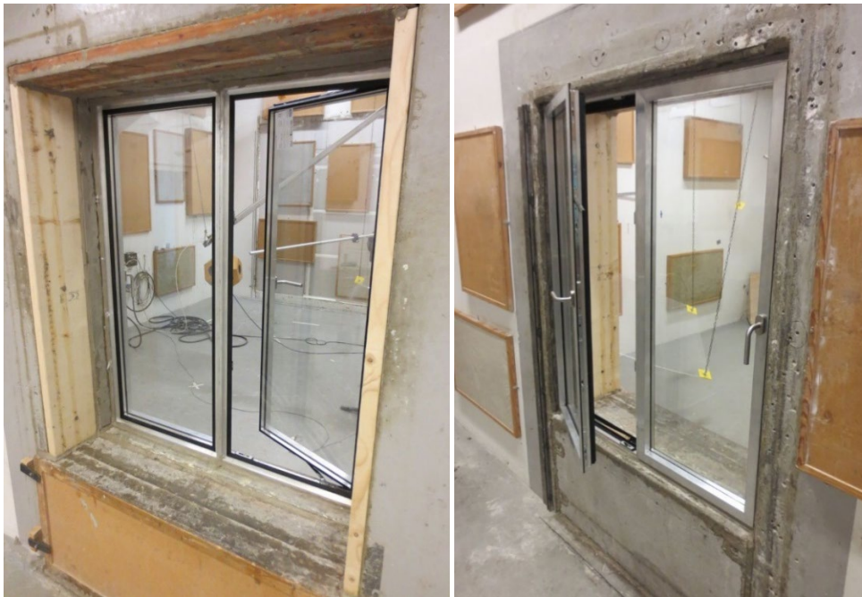
Illustration 8B. Photos of reference window: Single two-winged window shown from both inside (left photo) and outside (right photo).
