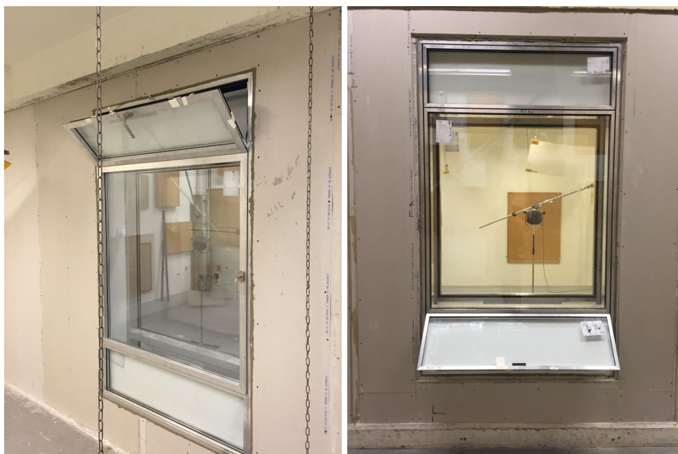
Illustration 7G. Left side: photo taken from the inside showing absorber lined on the vent and the glass on the opposite side of the vent. Right side: photo taken from the outside showing absorber lined on the vent and the glass on the opposite side of the vent.
