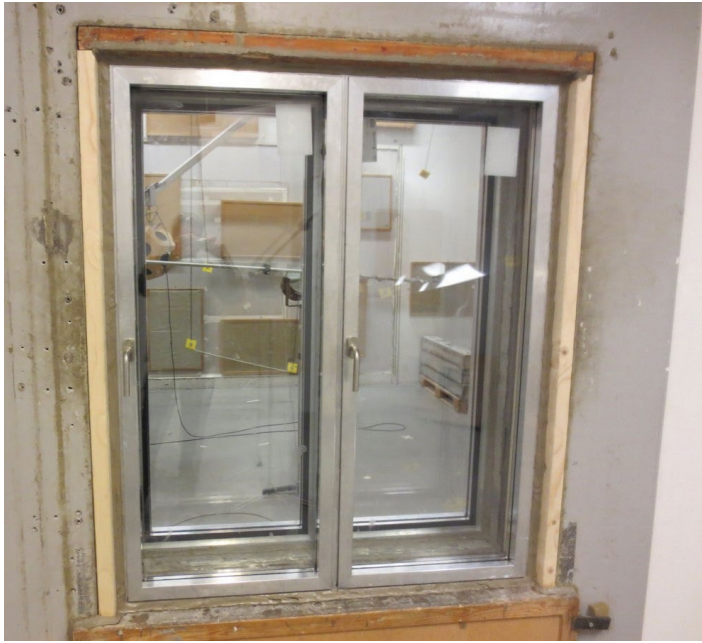
Illustration 8C. Photo of the closed double window seen from the inside.
