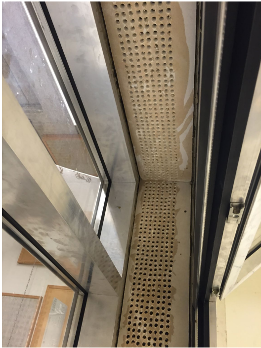
Illustration 7E. Photo of the window with 34.91 % perforated frame installed. The photo shows the upper corner.
