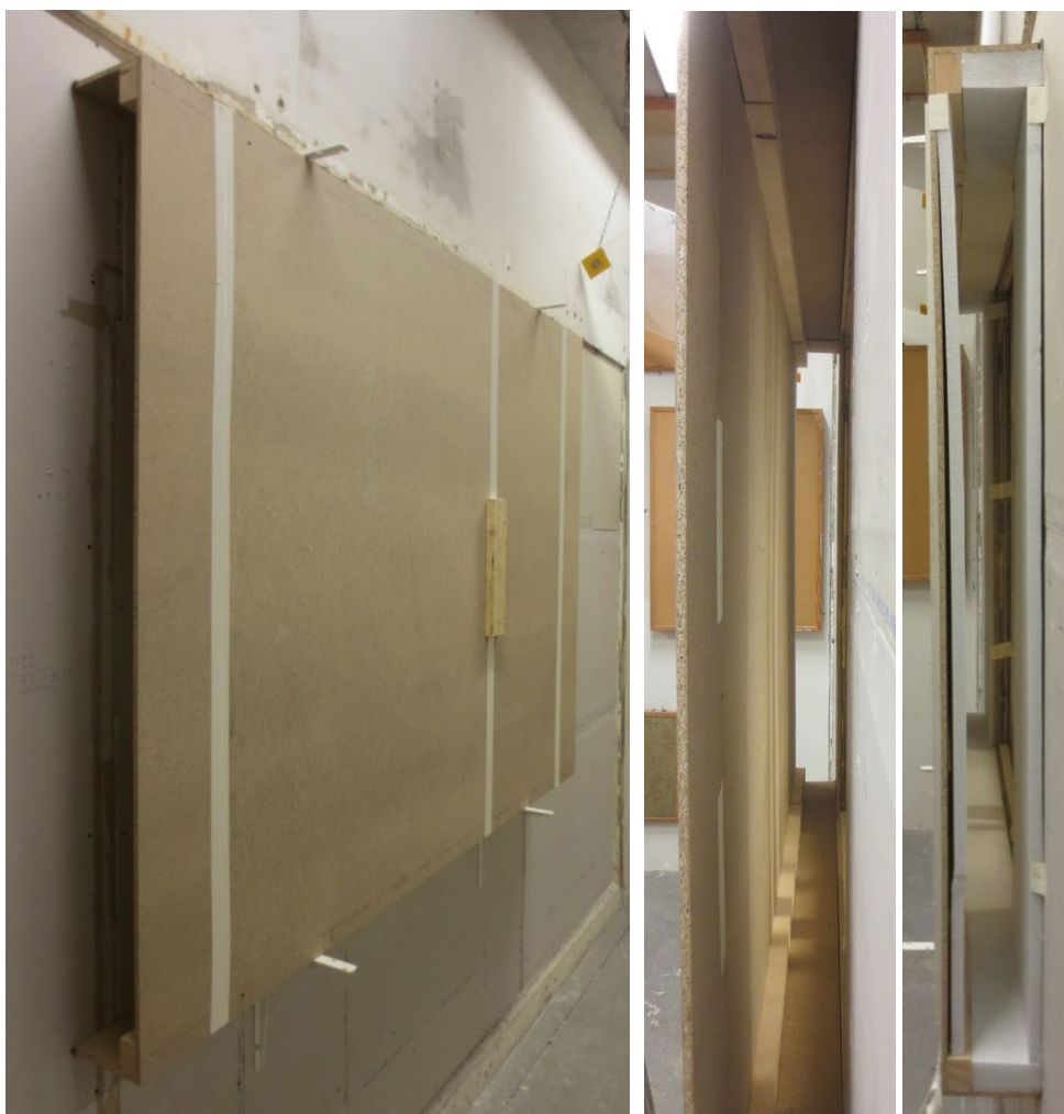
Illustration 9D. Photos of the actual implementation of mockup solution A. Left photo shows the extended version mockup solution A from the outside without added fiber gypsum. The middle photo is taken from one end and shows the construction without added absorber. The right photo is also taken from one end and shows the construction with added 20 mm absorber in the sides and 40 mm in top and bottom.
