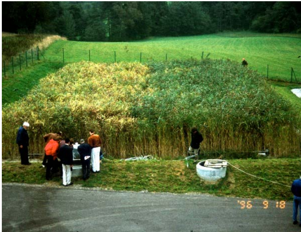
Vertical-flow constructed wetland system in Austria. The system contains two beds operating in parallel (Foto: H. Brix)
