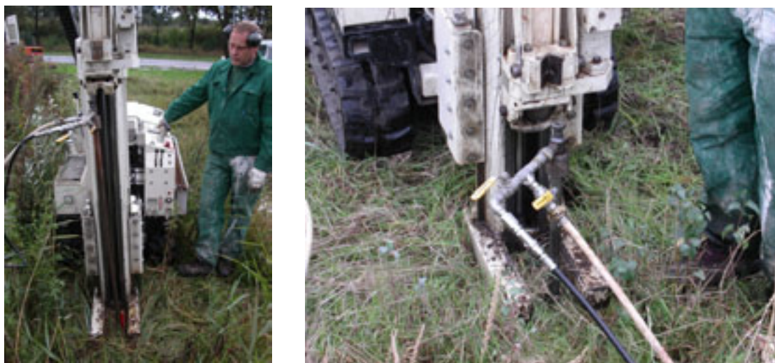
Figure 5. Direct injection of an electron donor. Left: the injection conus is pushed into the soil. Right: the electron donor is injected using a high pressure pump.
