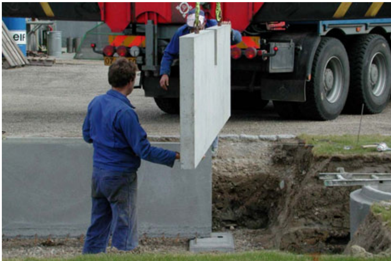
Figure 2. Building of the frame for the biobed. An excavation was made for both biobed and reservoir (see right). The concrete sides were brought in place, and the bottom was closed by concrete.
