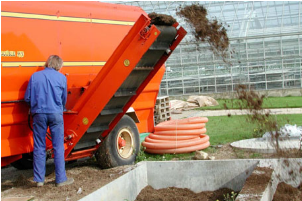
Figure 4. The biobed was filled with a mixture of chopped wheat straw (50%), sphagnum (25%) and soil from ploughlayer (25%). The mixing was performed in a feed mixer hired from a feedstuff business. Photo September 27 th 2001. Roll grass was placed on November 2001
