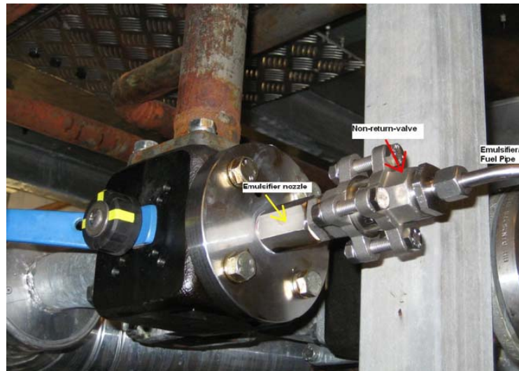
Figure 34 Emulsifier nozzle with non-return valve with injection of emulsifier into the bend on the fuel pipe.
