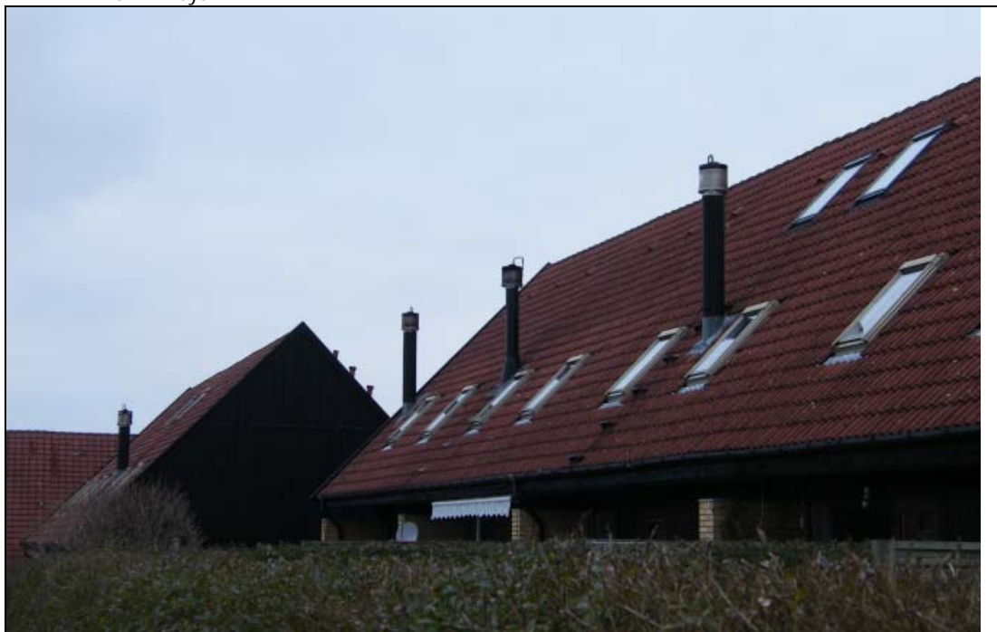
Figure 62. Photo showing the four chimneys mounted with APP electrostatic filters. The high voltage units were placed at ground level on the garden terraces below the chimneys.
