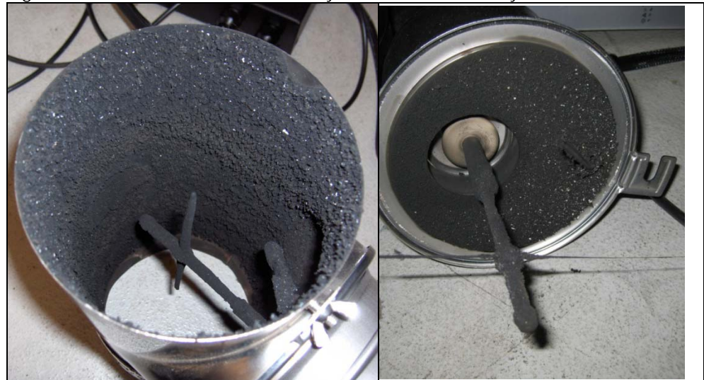
Figure 41. The Zumikon ESP after one day stove test and one day boiler test.
