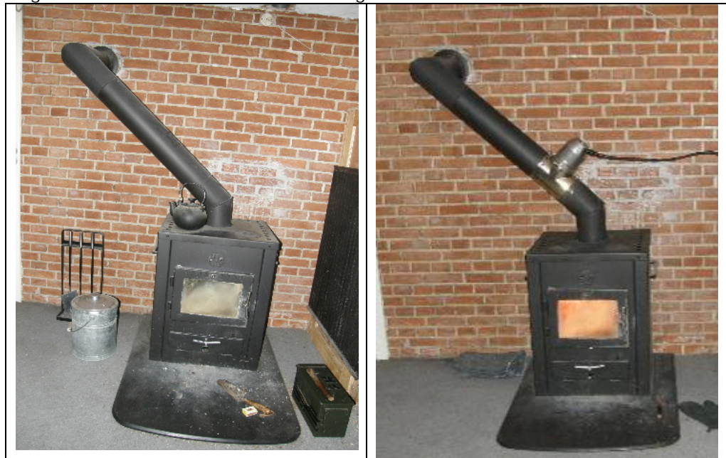
Figure 57. Stove before and after installing the Zumikon ESP
