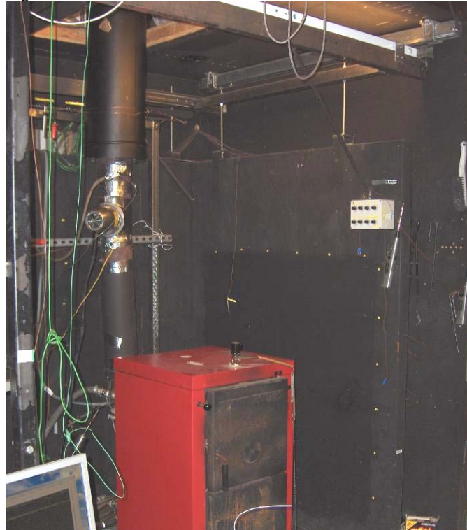
Figure 21. Viadrus wood boiler with Zumikon ESP
