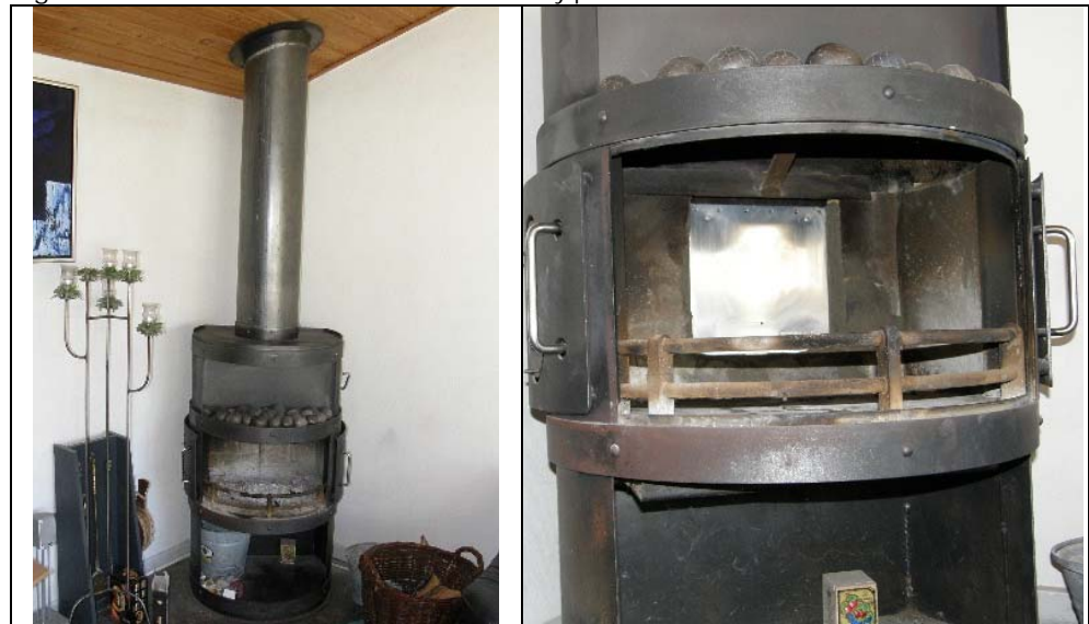
Figure 59. Rais stove from 1980 and the Ecoxy plate mounted inside on the back wall
