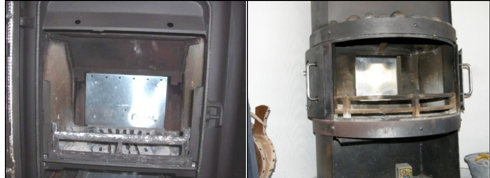
Figure 6. The Ecoxy retrofit plate for tertiary air supply mounted in two old stoves
