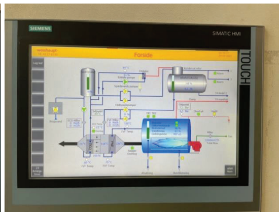
TH. Drift 6 tons kedel.
