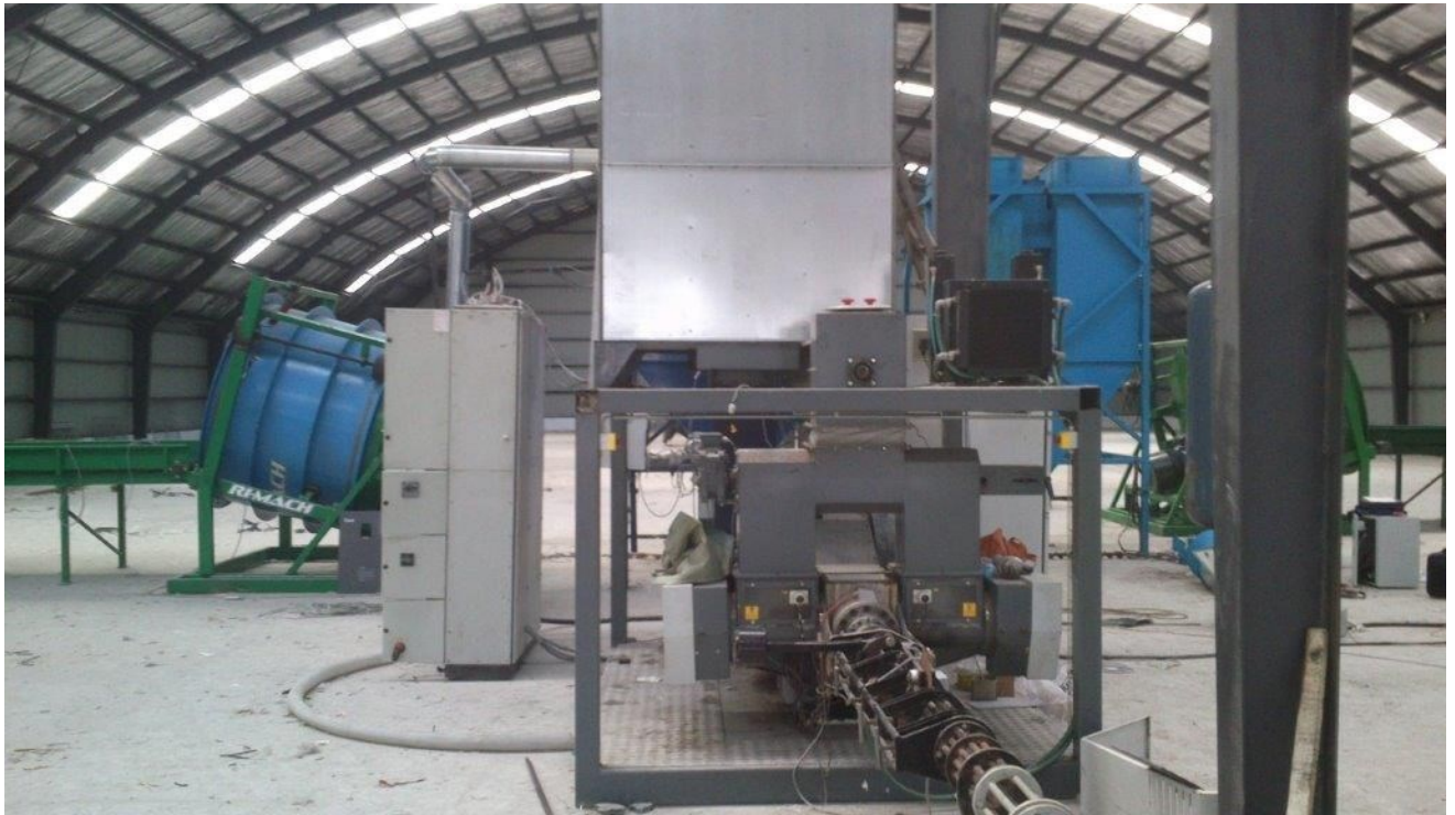
Installation of the briquetting product line, Harbin December 2018
