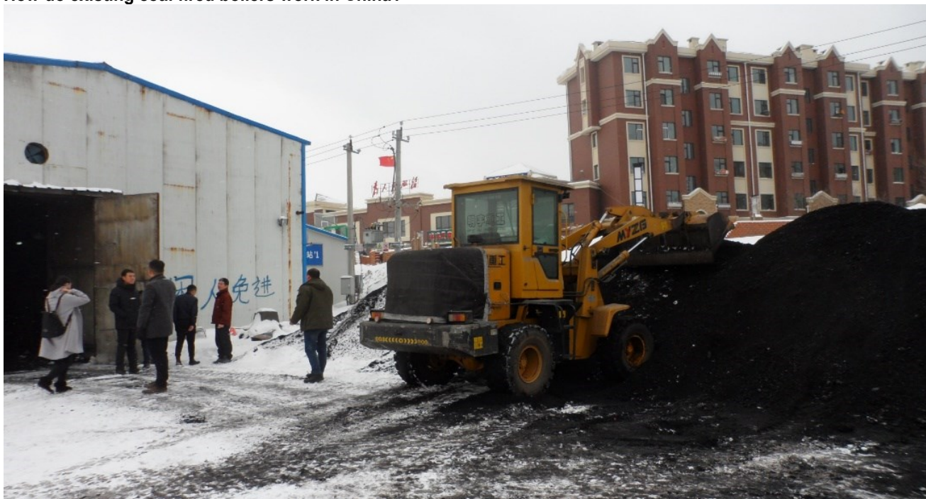
Inspection of a 7 MW coal fired boiler near dwelling blocks in Changchun, February 2017
