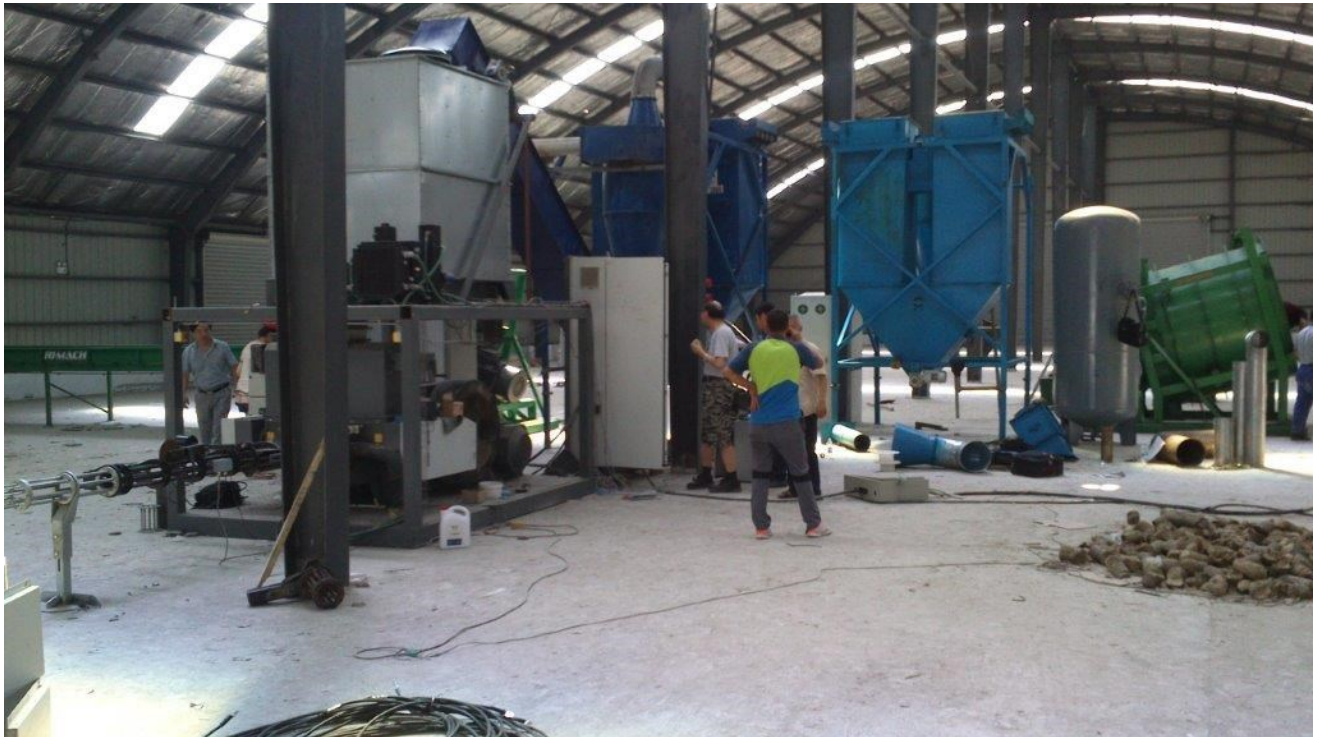
Lack of power from grid causes problems, Harbin December 2017
