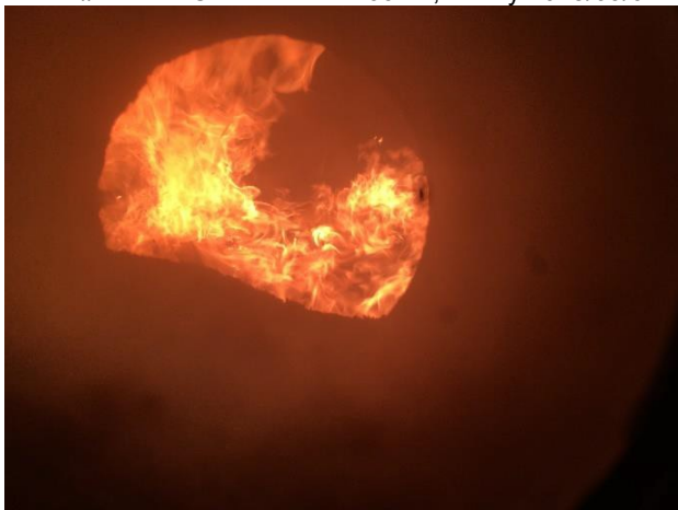
Photo # 2: Combustion with difficult fuel – ignition stopped at the right side of grate. Ignites at bottom of grate. At 11:29, Friday 2018/09/07
