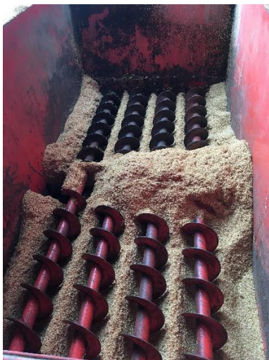
Fuel bin extraction system
