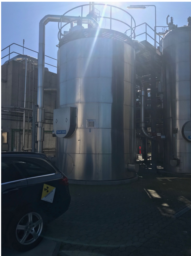
Thermal hydrolysis plant at Fredericia Central Treatment Plant
