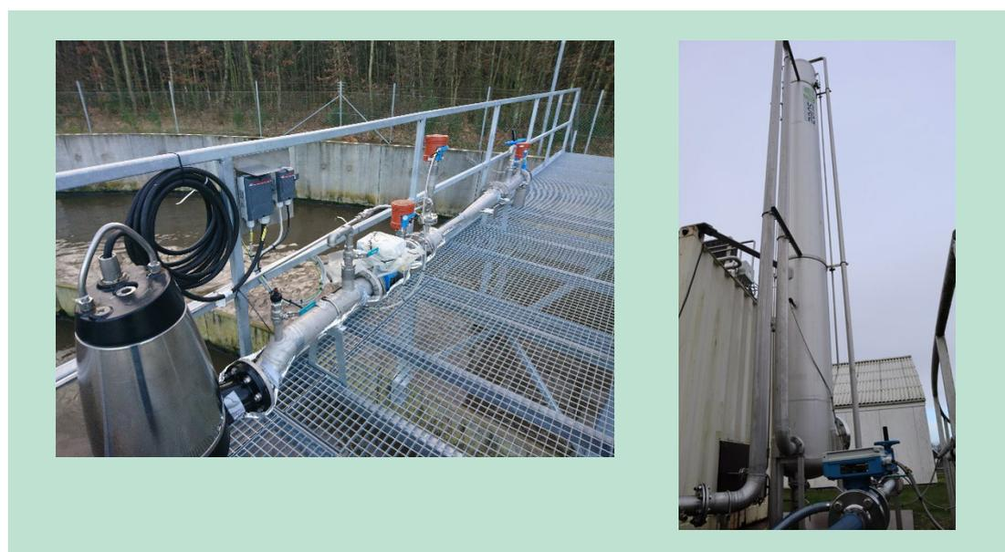
**FIGURE 9.** 2 points ozone injection - point 1: mixed liquor ozonation by venture ejector, Point 2: tertiary ozonation in ozone contact tank
