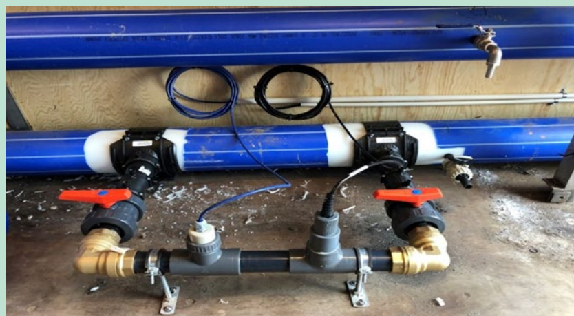
FIGURE 17. Conductivity and turbidity sensors installed in the pilot container.
