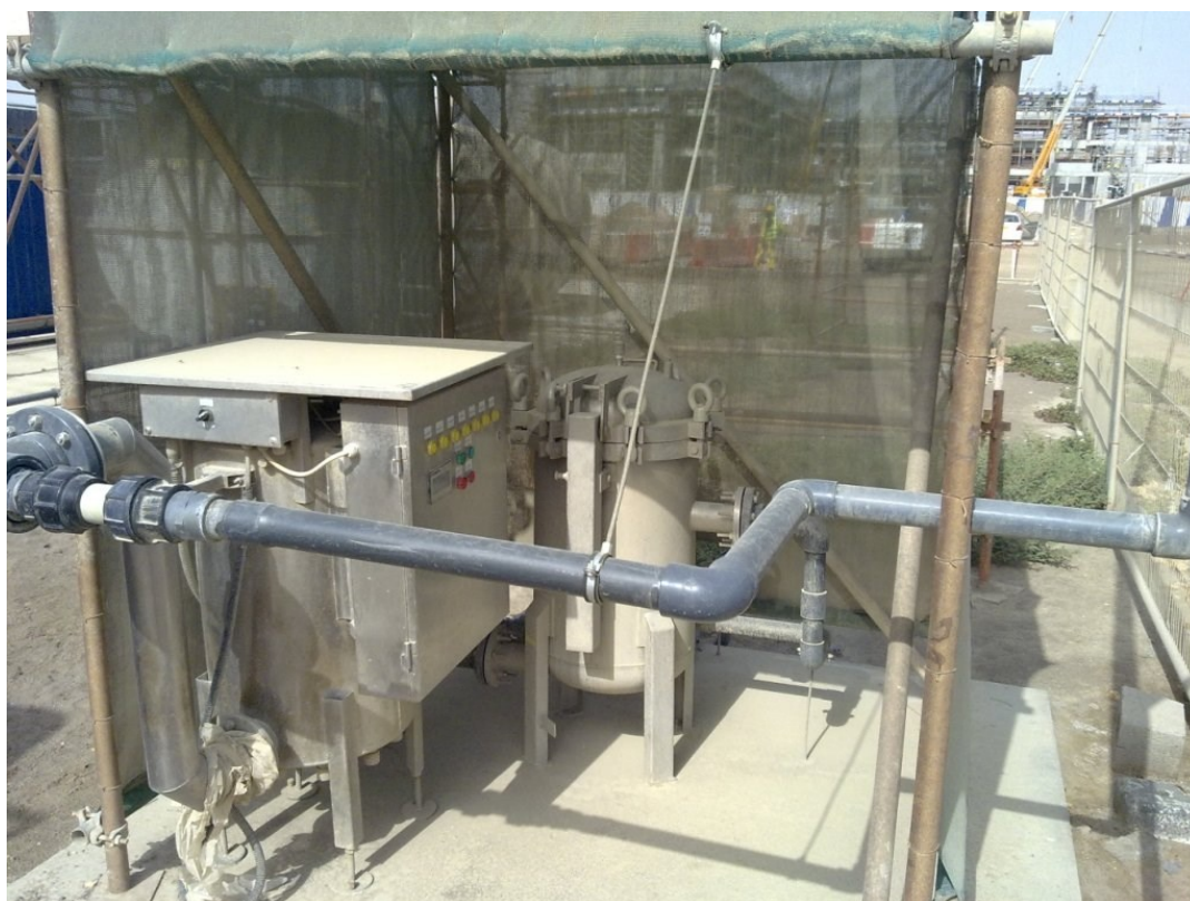
Figure 4.15 Biokube disinfection system installed after a traditional Biokube wastewater treatment installation in Oman. The disinfection system was equipped with a 10 µm bagfilter and UV (130 m 3 /d).
