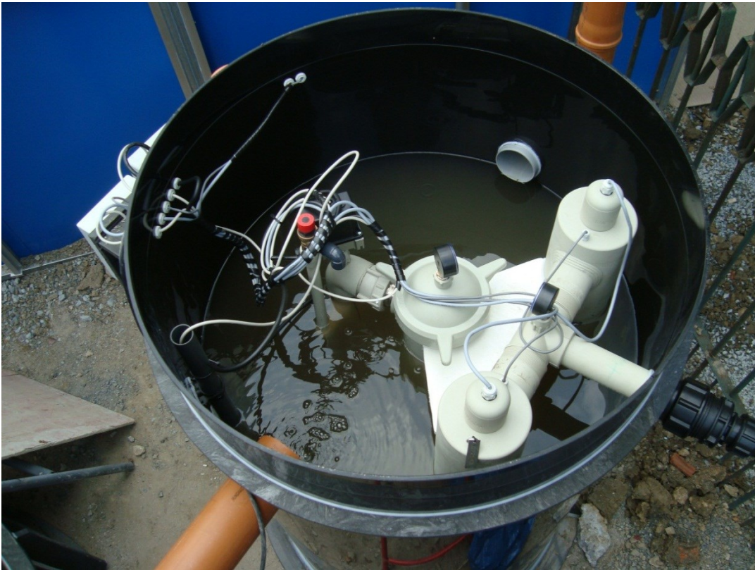
Figure 4.13 Disinfection tank in use just after start-up of the installation in Suzhou, China (November 2011)
