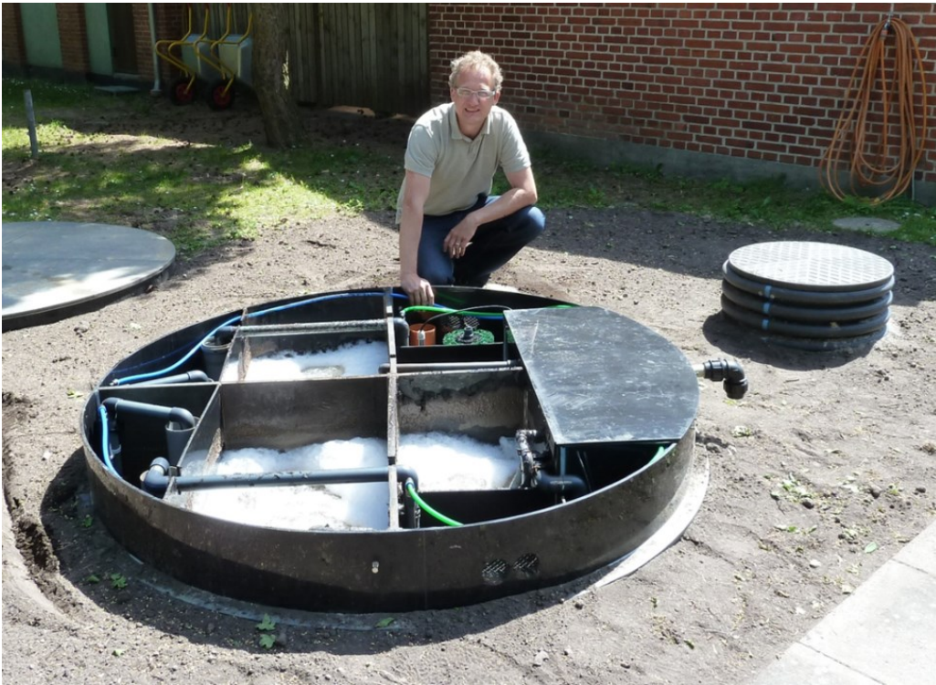
Figure 4.5 Installation of a Biokube Mars 3000 in the ground (photo taken of an installation in Denmark similar to the experimental setup in China)
