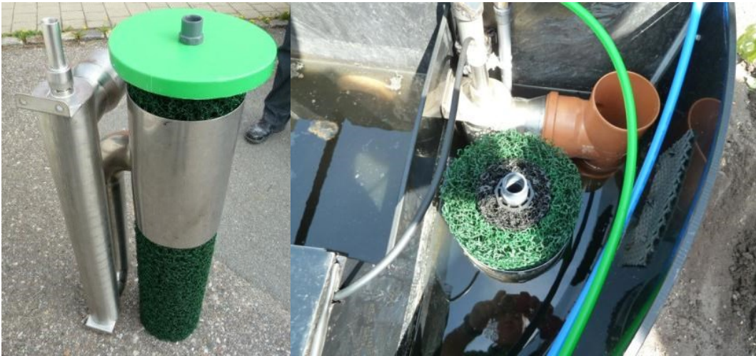
Figure 4.8 Pre-filtration unit installed in a Biokube Mars 3000 for extra fine purification of the wastewater
