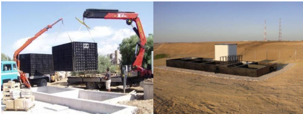
Figure 3.4 Installation of a Biokube wastewater treatment plant. Installation of the biological part of the wastewater treatment plant and pre-sedimentation typically takes one day after the concrete tanks have been prepared
