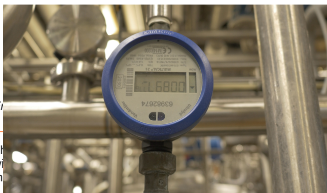
Water meter installed in Thise Dairy (copyright photo Thise Dairy)
