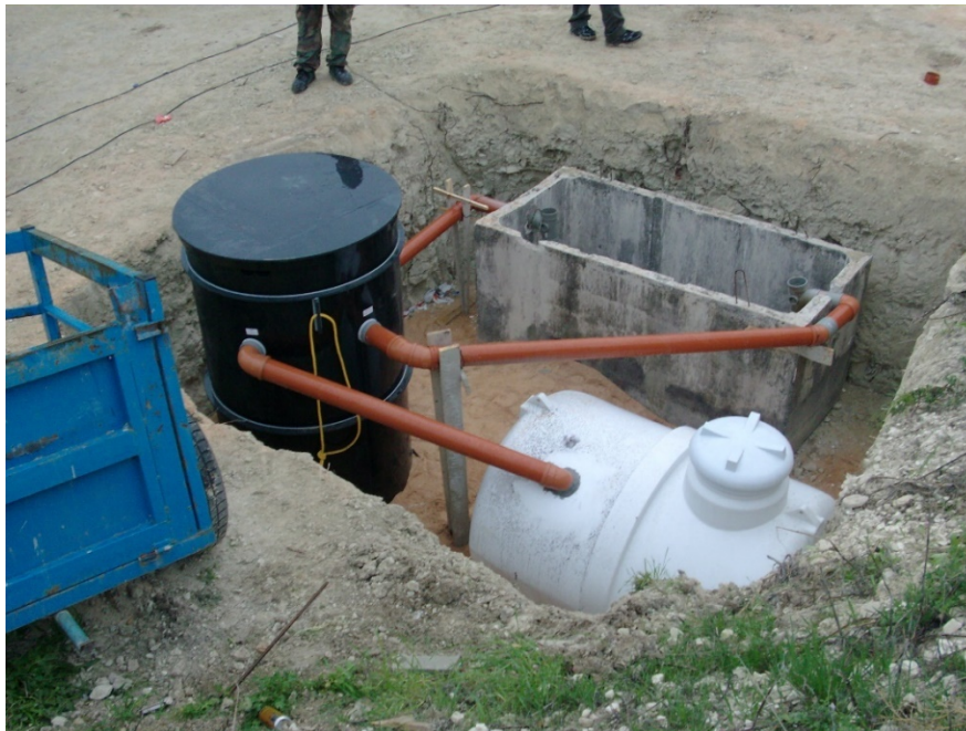
FIGURE 18 Illustration of system setup for reuse for irrigation. You see
