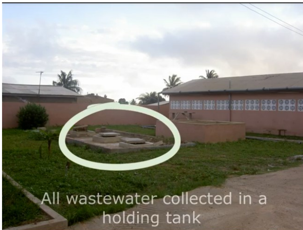
FIGURE 40. With very little of the wastewater treated at central plants in Accra, most wastewater is collected in storage tanks. The picture shows a storage tank at a facility with public toilets.
