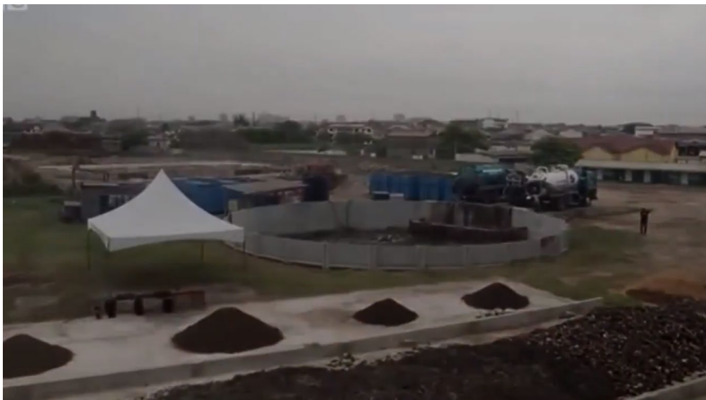
FIGURE 42. Treatment system installed in Accra, Ghana. Sewage from the sludge trucks is deposited in the large concrete tank (H = 5 m / Ø = 22 m) from where it is processed. The system can handle 140 sludge trucks per day. Equivalent to wastewater from over 70.000 PE.
