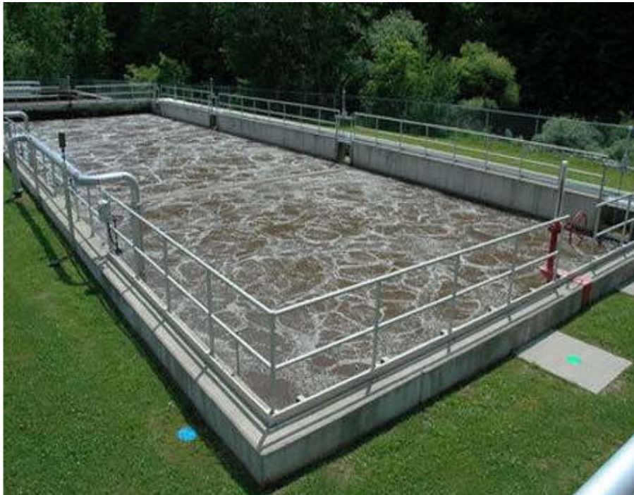
FIGURE 5. Treatment chamber in an activated sludge system.
