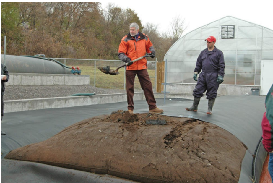
FIGURE 36. After a few weeks the sludge in the GeoTube will have a dry content of over 70% giving the possibility of easy reuse or disposal.
