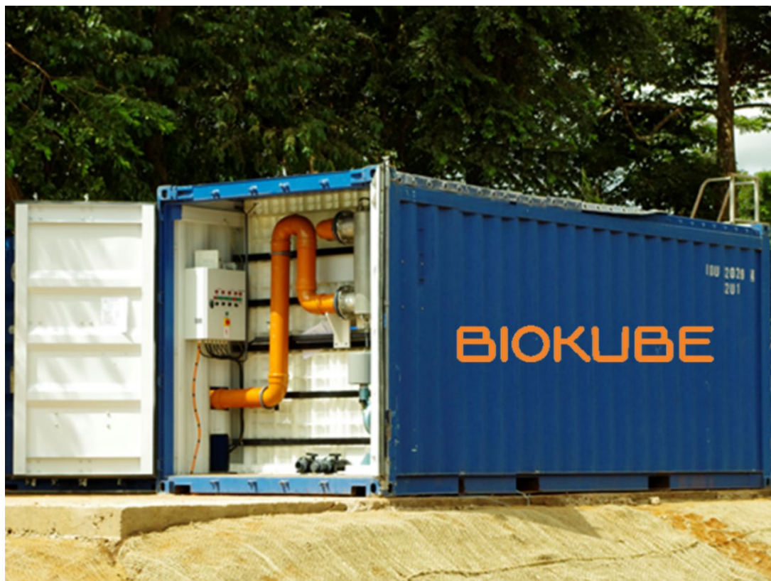
FIGURE 50. Biokube 20 foot container wastewater system at work camp in Guinea. The aluminum “tube” on the right side is the UV lighting system for removing all pathogen bacteria.
