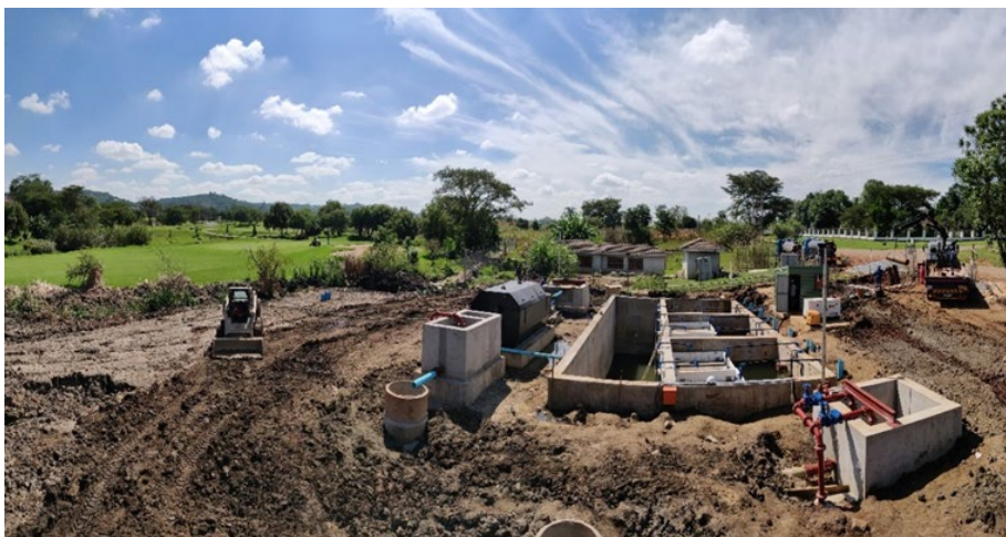
FIGURE 19. BioKube system under installation at golf course in Harare, Zimbabwe. The
