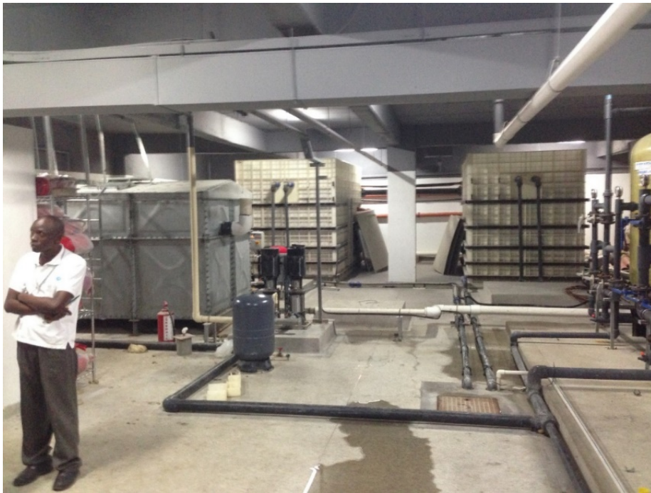
FIGURE 22. BioKube system installed in the basement of a luxury hotel in Mombasa, Kenya. The wastewater treatment is the white boxes. Treated water is stored in the steel tanks and the water reused for toilet flushing and watering the green areas around the hotel.
