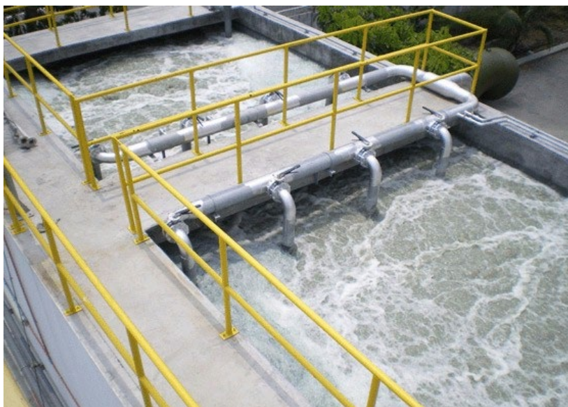
FIGURE 11. An MBBR system in operation. You can see the floating media
