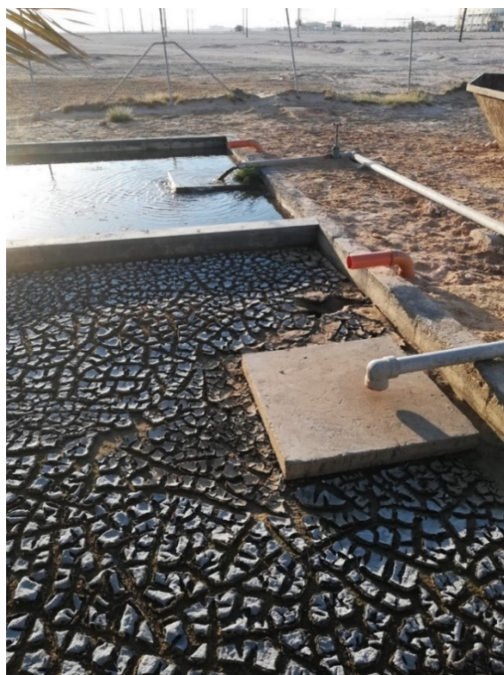
FIGURE 28. Sludge drying bed in operation in Oman by a BioKube system. It uses simple evaporation to
