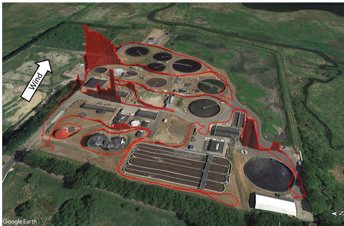
Figure 3 – On-site screening of methane concentrations started at 11:39 on 21/08/2019. Concentrations were recorded at 2 m above ground. Methane concentrations are showed above background level (1.94 ppm) and multiplied by a factor of 20 in order to be displayed on the map. The North direction is shown at the bottom right of the Figure.
