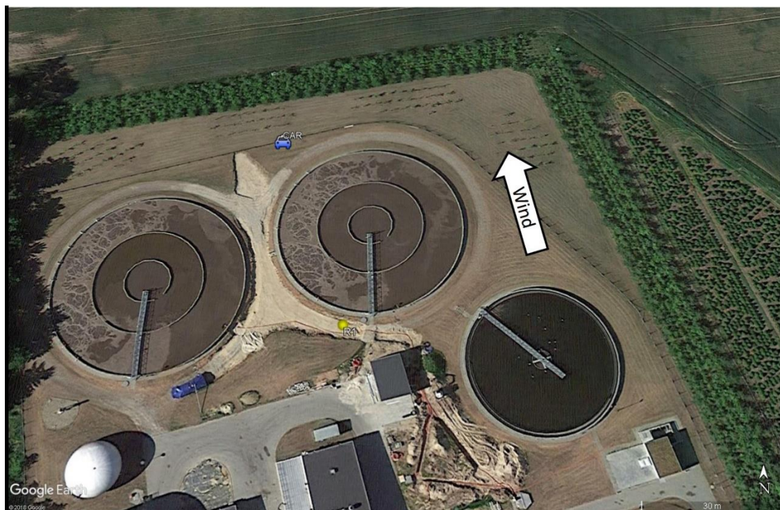
Figure 5 – Location of the tracer gas (acetylene) release and the position of the mobile measurement platform during the application of the static tracer gas dispersion method at one of the activated sludge reactors on 13/06/2019. Tracer release is marked with a yellow dot (R1), while the mobile measurement platform position is marked with a blue car. The North direction is shown at the bottom right of the figure.
