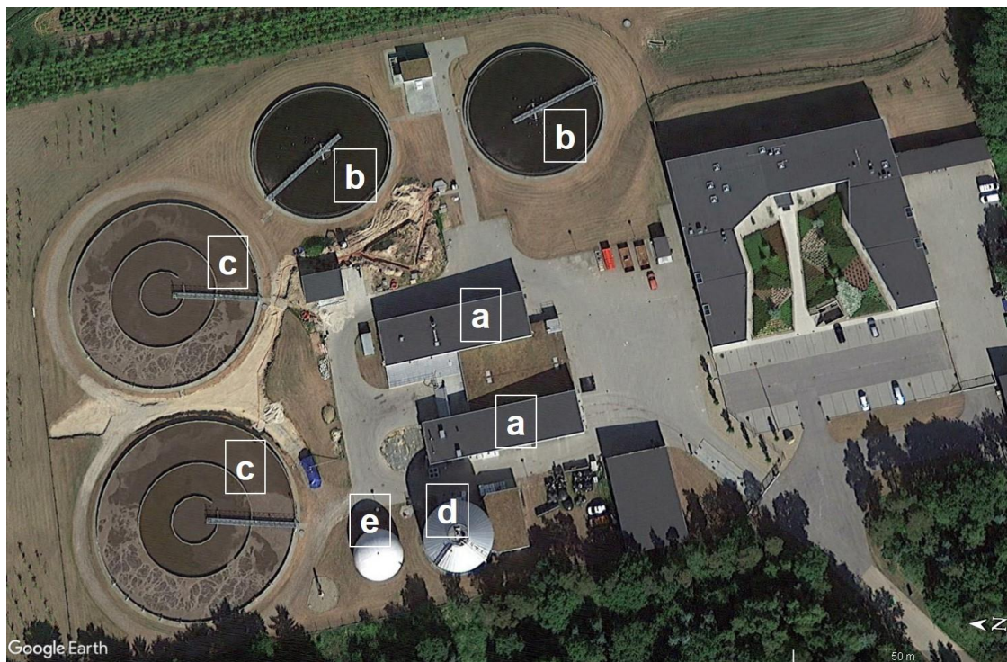
Figure 1 – Location of main process units at Mariagerfjord wastewater treatment plant in Hadsund. a) Indoor treatments: mechanical pretreatments, sewage sludge and biosolids dewatering, and biosolids storage; b) Settlers; c) Activated sludge reactors; d) Anaerobic digester; e) Gas holder. Notice the North direction at the bottom right of the figure.
