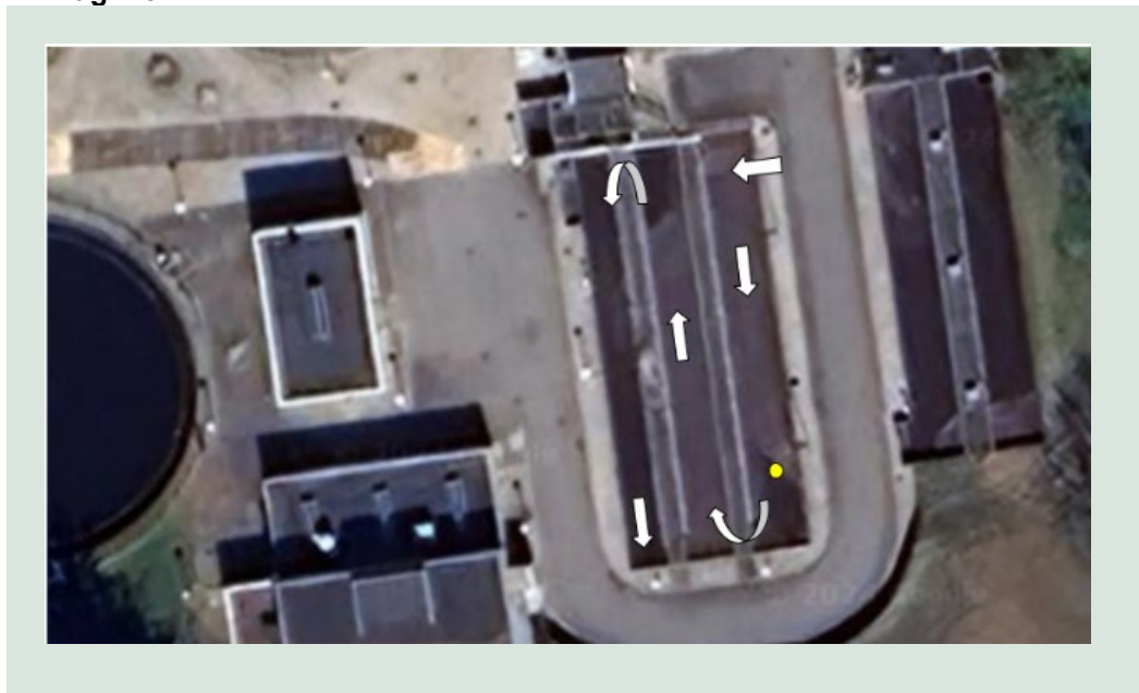
Figure B6. Case C: Stavsholt treatment plant (Novafos) – a plug flow system
