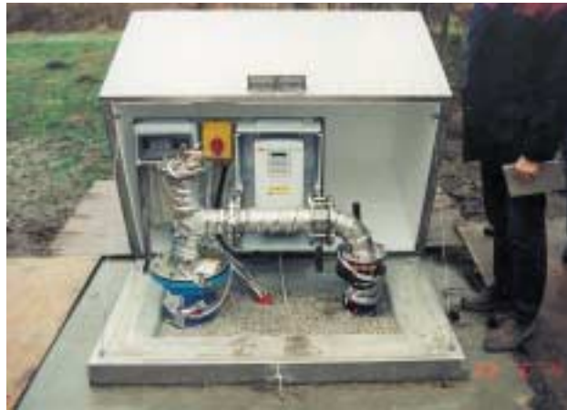
Figur 34 Installation af dykpumpe
