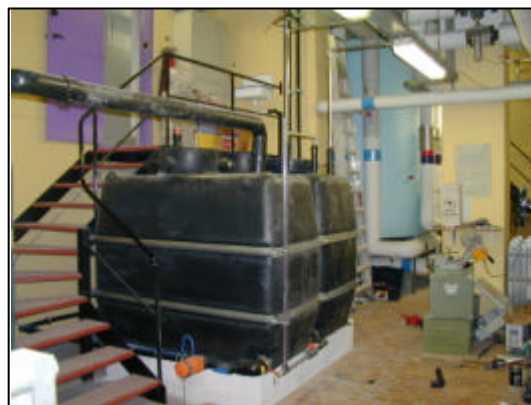
Figur 2.7: Sedimentationstanke i varmecentral
