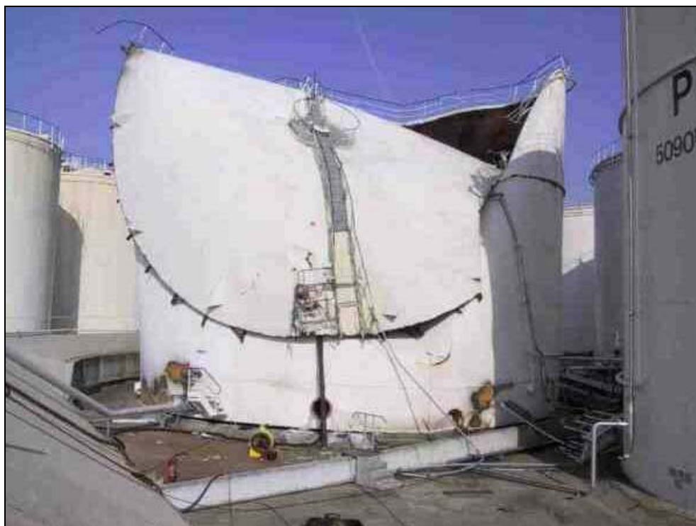
Figur 6.9 Eksploderet tank i Lespinasse /ref. 4/.
